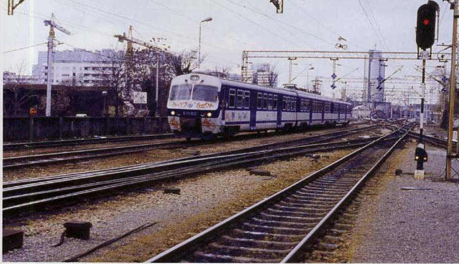
Suburban rail operations with EMU type 6111. Suburban rail services in Zagreb have reached a good level, similar to other European capitals. Financing and funding procedures of services, unfortunately, have not yet reached best practice. Photo: Wolf-Dietrich Geitz.
